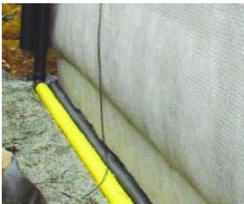
**Figure 5** Example of a land drain. Courtesy of Safeguard Europe
