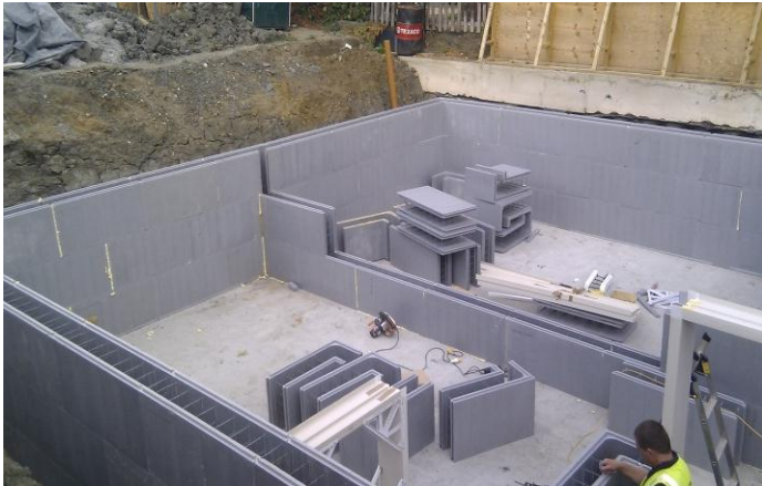
Cheltenham basement currently under construction
